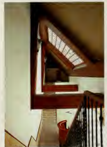
The Hall of Deputies's pyramidal shape is expressed in the entry foyer, where monumental stairs leading to the main chamber help create a strong transitional experience for visitors. Photograph: Fernando Revollo
